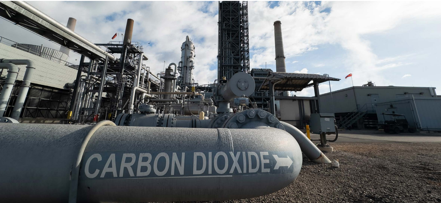
The Petra Nova facility that captures CO 2 from post-combustion flue gas at NRG’s W.A. Parish coal power plant in Texas, USA. Image courtesy of Petra Nova facility owner, ENEOS Xplora Inc.
